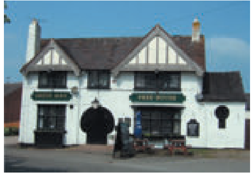
Under threat; Note the 'keyhole' entrance and window and the Bass lantern sign
