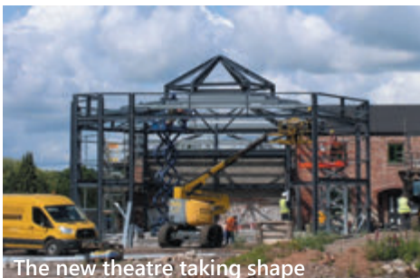
The new theatre taking shape
